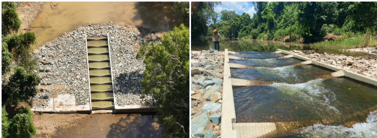
Figure 3. Overview of Carmila Gauging Weir fishway after completion prior to its first flow (left) and with the low flow trapezoidal ramp engage during a low flow (right).
