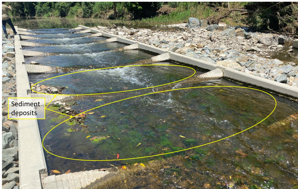
Figure 14. Sediment deposits within pools of the low flow channel at Carmila Gauging Weir fishway.
