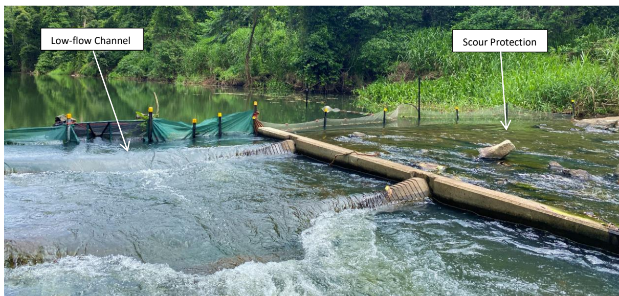
Figure 5. Trapping of the low-flow channel and scour protection of the northern bank scour protection.
