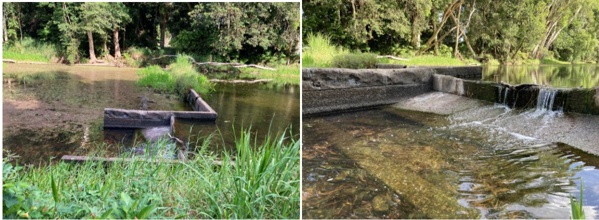
Figure 2. Carmila Gauging Weir prior to the fishway construction.
