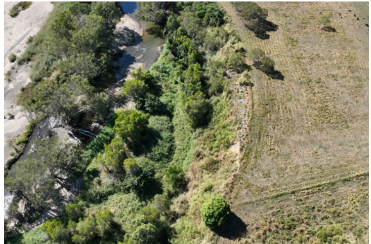
Figure 1 - Reef Catchments’ Glassons site erosion extent before works.
