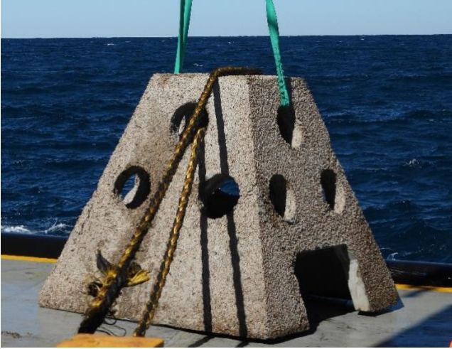
Photo (above): Installation of Habitat Reef Module
