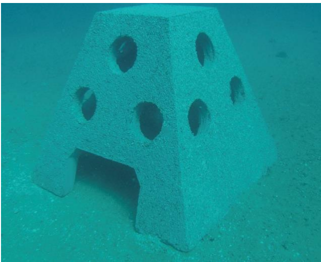
Photo (above): Installed Habitat Reef Module (photo credit: Catchment Solutions)
