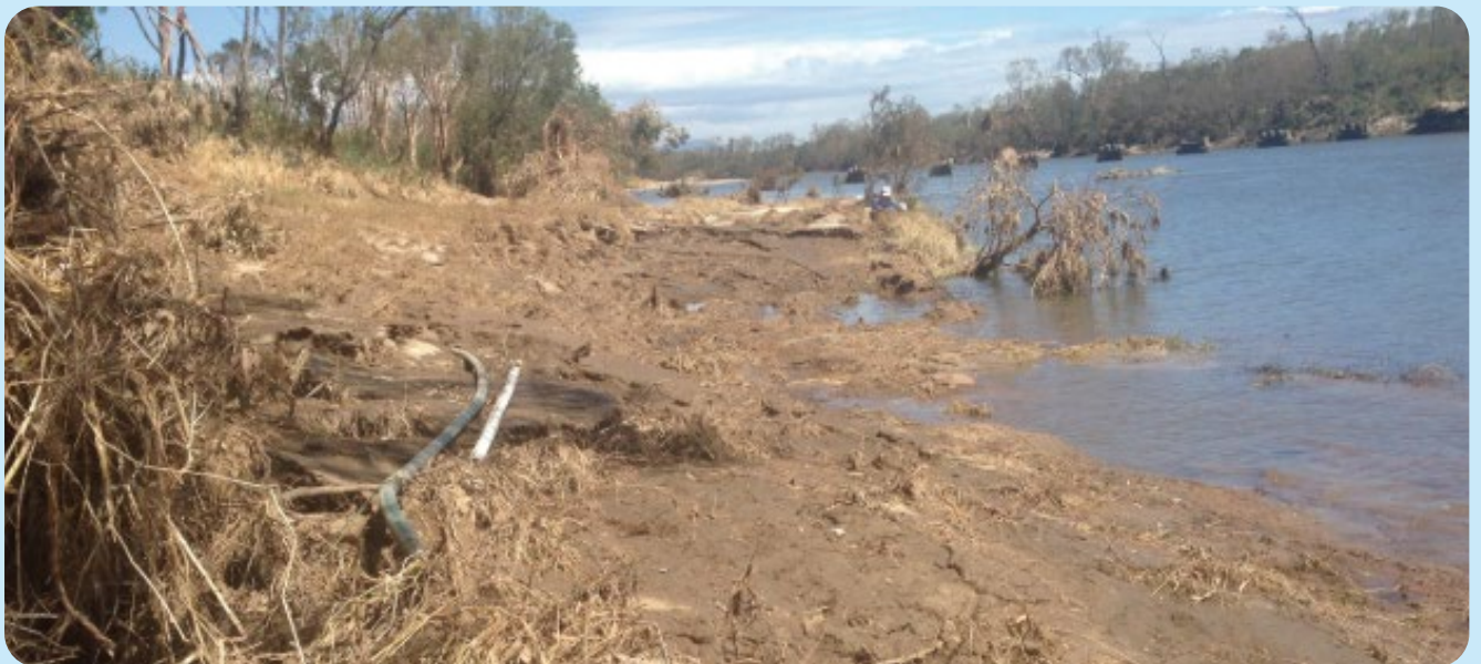
Figure 15: Bank erosion and loss of water monitoring infrastructure on the O'Connell River.
