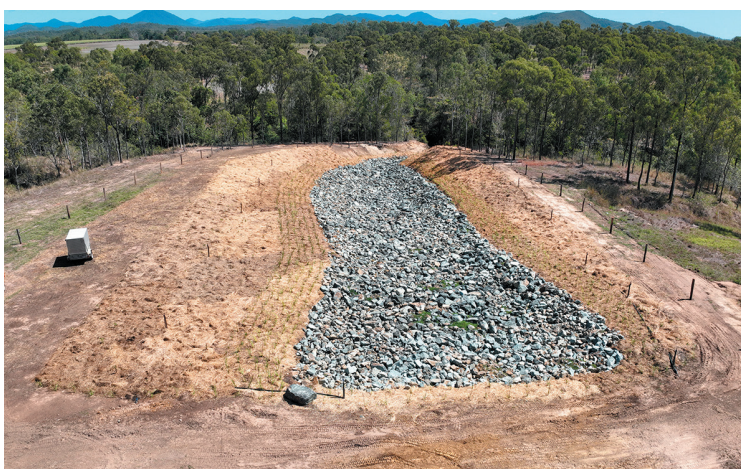
Figure 14 - A repaired gully on a landholder's property (Reef Catchments, 2023)
