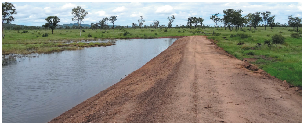
Figure 13 - An example of a diversion bank on grazing property (Smith, 2018)
