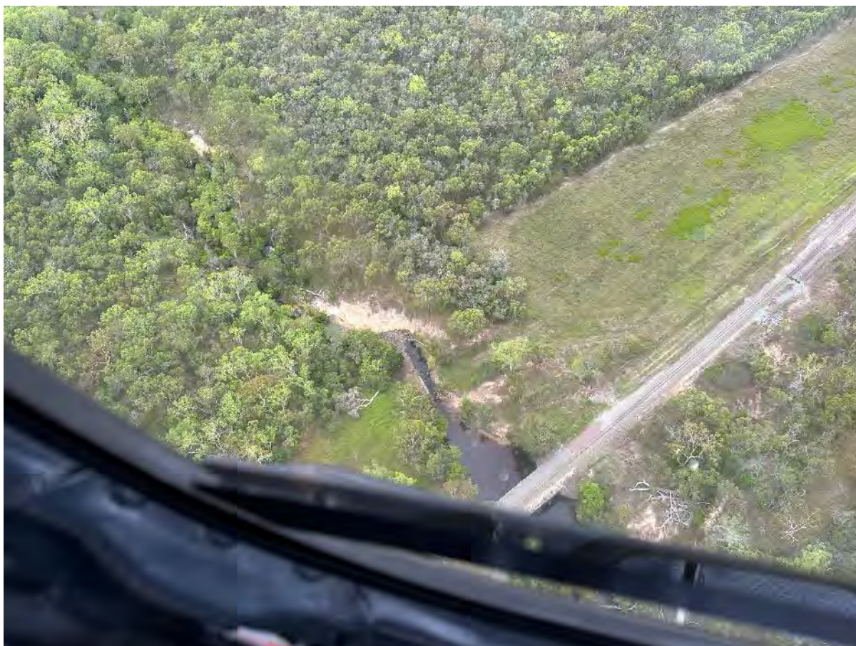
Figure 98. Photo of feature 516 along Kelly Creek downstream of a rail crossing
