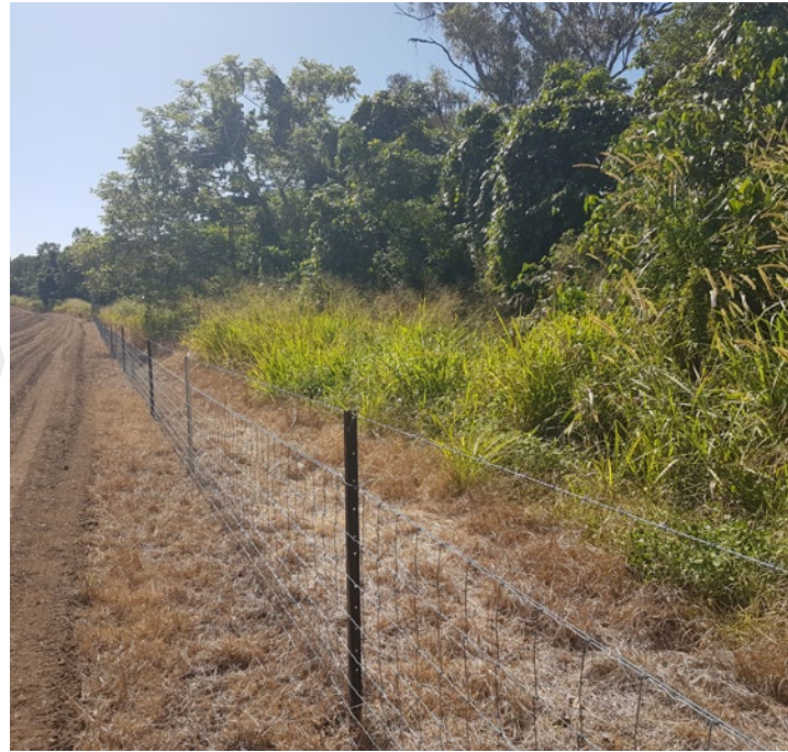
Figure 4 - An example of Feral Pig exclusion fencing installed in the O'Connell Basin.
