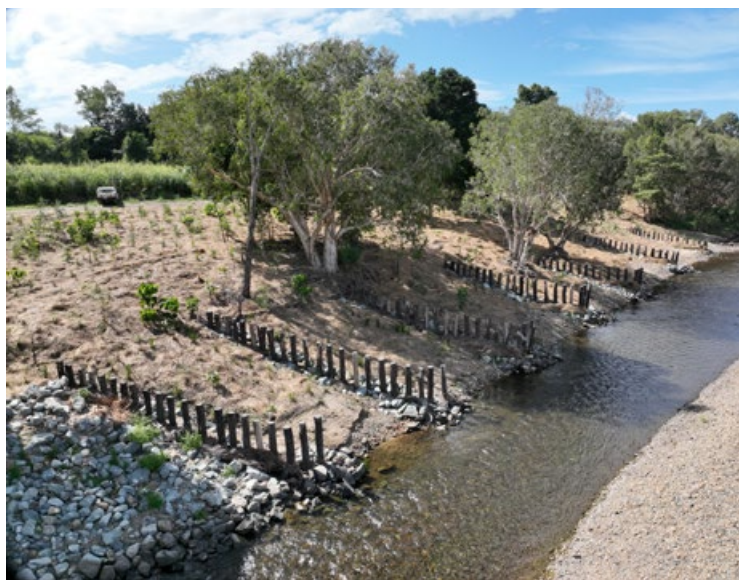
Figure 5: SB006 a RTVII streambank pile field remediation site installed along the O'Connell River
