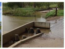
Figure 17. The floodgates on pond 2 of Marklands Wetlands (left), typical habitat within the wetland complex (middle), and the cone fishway constructed in 2015 on the large Pond 3 (right).
