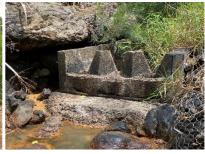
Figure 15. Flaggy Rock Creek Weir in 2007 (left) and 2021 (mid). Extensive vegetation has established on the crest of the weir which would assist with fish passage when flow is overtopping the crest. During low flows fish passage is significantly impacted as the fishway outlet is 0.5 m above the tailwater level.
