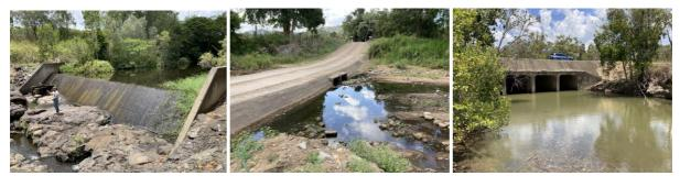
Figure 4. Examples of low (left), medium (mid) and high (right) passability fish barriers.
