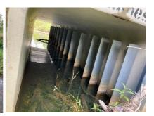
Figure 21. Streeters Rd causeway on Carmila Creek, prior to the upgrade (left) and after replacement with a fish friendly causeway (mid). Note the combine aperture of the culverts and floor depth. Vertical baffles were also installed on the outer cell walls to reduce velocity during higher flows (right).
