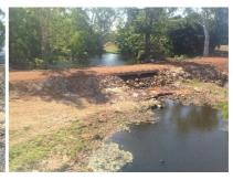
Figure 23. Recently constructed/upgraded causeways which do not meet current statutory requirements for fish passage in Queensland waterways.
