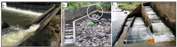
Figure 2. Examples of early fishways based northern hemisphere designs exhibiting hydraulic conditions greater than the swimming abilities of most native freshwater fish species. a. Denil fishway on Luscombe Weir (Albert River, QLD). b. Pool and weir fishway located on the Bremer River (Berrys Weir). The exit of this style of fishway has a 600 mm high drop and velocities during base flows of 3.3 m/sec. c. Pool and weir fishway located on Marian Weir (Pioneer River, QLD).
