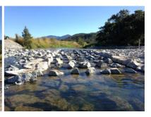
Figure 22. Clews Rd causeway on Murray Creek, prior to the upgrade (left) and after the causeway was rebuilt following flood damage (mid). Note that all flows pass over the causeway and fish passage is provided by the full width rock ramp on the downstream side. During high flows the entire fishway is engaged and under low flow conditions the flow is concentrated to the central pool and ridge low flow channel (right).
