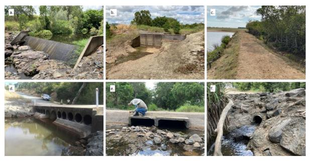
Figure 1. Barrier structures: a. irrigation supply weir (McGregor Creek), b. tidal floodgates (Constant Creek Tributary) c. Earth bund (Constant Creek floodplain), d. Pipe culvert causeway (Daintry Creek), e. box culvert causeway (Carmila Creek), f. Perched pipe culvert causeway (Gibson Creek).
