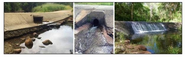
Figure 3. Left to right: Culvert causeway displaying a water surface drop, shallow water surface (through culvert and on apron) and velocity barrier (during medium- high flow conditions) exacerbated due to a culvert diameter <60% of stream width; Pipe causeway displaying velocity and behavioural barriers (insufficient lighting in pipe) and water surface drop barrier.
