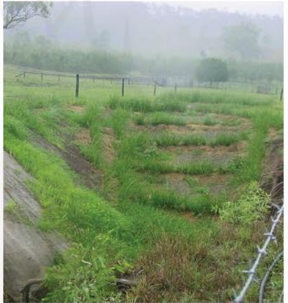
Vetiver stabilisation & protection 2 months
