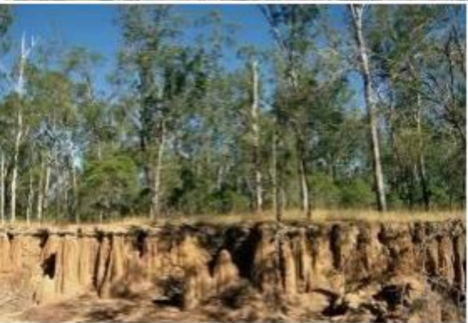
Photograph 47. Severe gully erosion on Ulogie soil due to the highly dispersive subsoil
