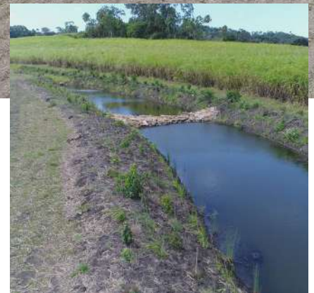
Above: The constructed chain of ponds designed to capture contaminants.
