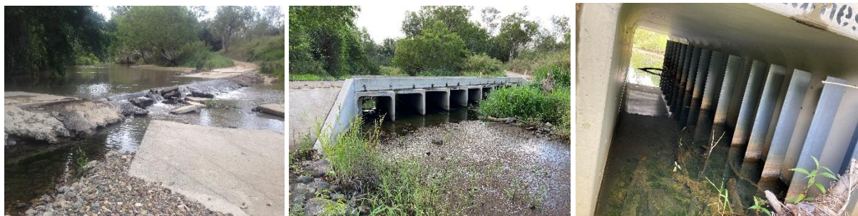
Figure 21. Streeters Rd causeway on Carmila Creek, prior to the upgrade (left) and after replacement with a fish friendly causeway (mid). Note the combine aperture of the culverts and floor depth. Vertical baffles were also installed on the outer cell walls to reduce velocity during higher flows (right).
