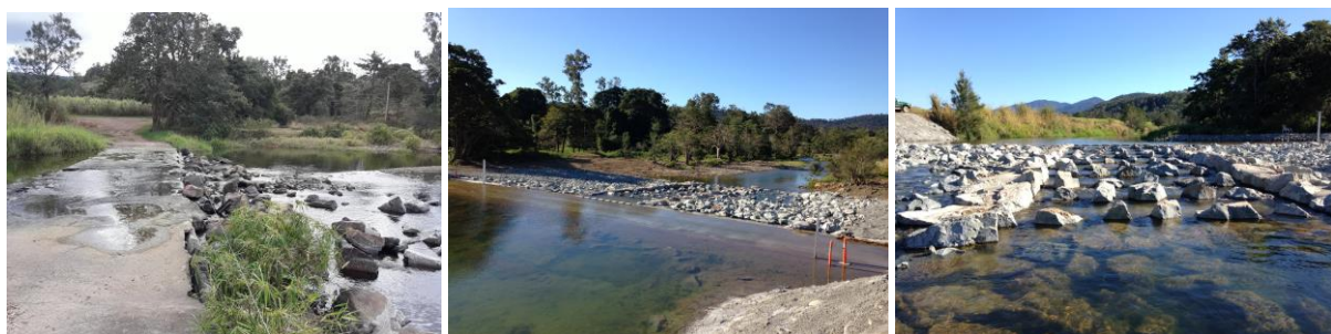
Figure 22. Clews Rd causeway on Murray Creek, prior to the upgrade (left) and after the causeway was rebuilt following flood damage (mid). Note that all flows pass over the causeway and fish passage is provided by the full width rock ramp on the downstream side. During high flows the entire fishway is engaged and under low flow conditions the flow is concentrated to the central pool and ridge low flow channel (right).
