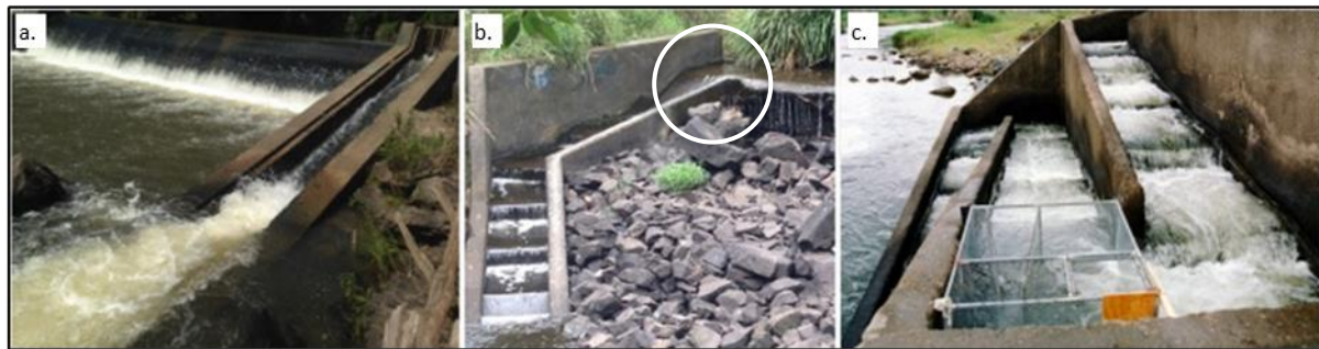
Figure 2. Examples of early fishways based northern hemisphere designs exhibiting hydraulic conditions greater than the swimming abilities of most native freshwater fish species. a. Denil fishway on Luscombe Weir (Albert River, QLD). b. Pool and weir fishway located on the Bremer River (Berrys Weir). The exit of this style of fishway has a 600 mm high drop and velocities during base flows of 3.3 m/sec. c. Pool and weir fishway located on Marian Weir (Pioneer River, QLD).
