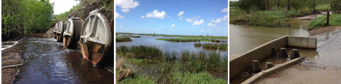
Figure 17. The floodgates on pond 2 of Marklands Wetlands (left), typical habitat within the wetland complex (middle), and the cone fishway constructed in 2015 on the large Pond 3 (right).
