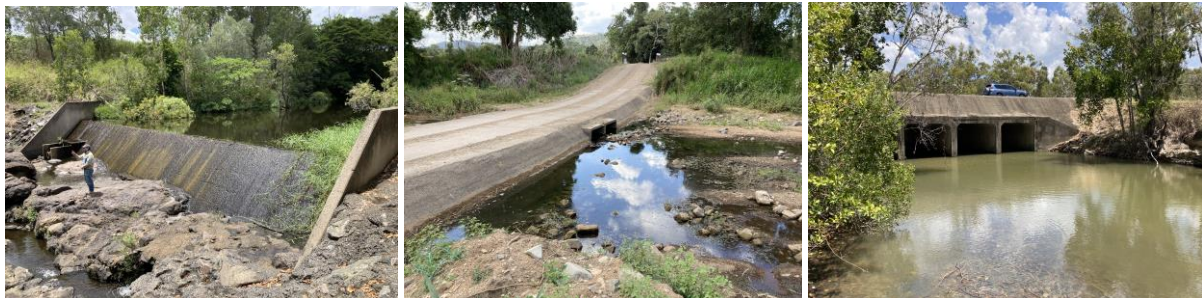
Figure 4. Examples of low (left), medium (mid) and high (right) passability fish barriers.
