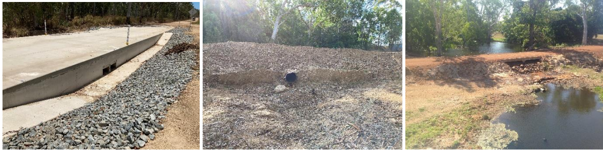
Figure 23. Recently constructed/upgraded causeways which do not meet current statutory requirements for fish passage in Queensland waterways.
