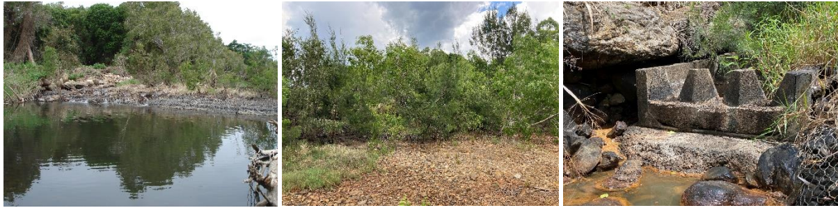
Figure 15. Flaggy Rock Creek Weir in 2007 (left) and 2021 (mid). Extensive vegetation has established on the crest of the weir which would assist with fish passage when flow is overtopping the crest. During low flows fish passage is significantly impacted as the fishway outlet is 0.5 m above the tailwater level.
