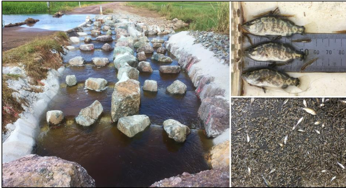
Figure 25. A rock ramp fishway constructed to remediate a road causeway (water surface drop) on Tedlands wetlands in Koumala, central QLD (left). Young of the year barramundi recruits captured successfully ascending the fishway during post-const construction monitoring (top right). This is the typical size of juvenile barramundi undertaking life-cycle dependant migrations from saltwater to freshwater. Thousands of juvenile empire gudgeon (and a few barramundi) recorded in a single trap set successfully ascending the fishway (bottom right). These empire gudgeon and barramundi were migrating from saltwater to freshwater.
