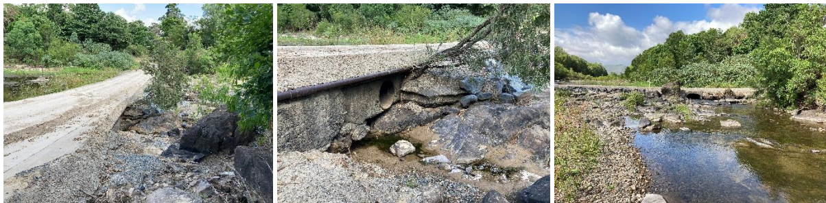
Figure 14. Staffords Rd causeway on the O'Connell R. looking west across the causeway (left) and showing the small pipe (mid) and box (right) culverts incorporated into this structure.
