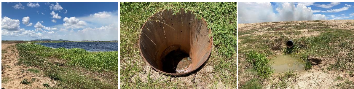
Figure 18. Looking across the dam wall (left) of Thompson Creek upstream wetland and the inlet (middle) and outlet (right) of the stand pipe which currently passes low flows.
