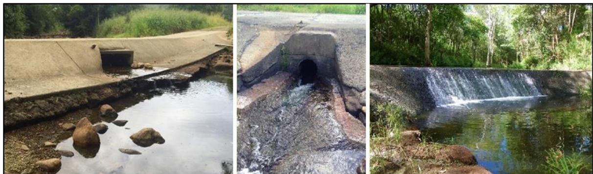
Figure 3. Left to right: Culvert causeway displaying a water surface drop, shallow water surface (through culvert and on apron) and velocity barrier (during medium- high flow conditions) exacerbated due to a culvert diameter <60% of stream width; Pipe causeway displaying velocity and behavioural barriers (insufficient lighting in pipe) and water surface drop barrier.
