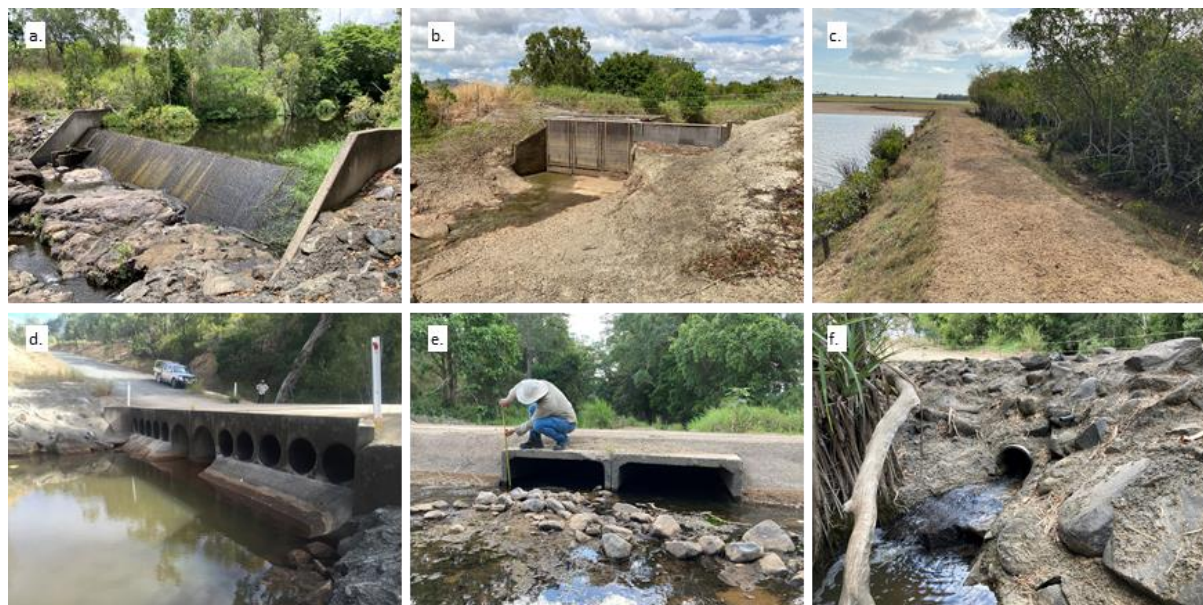
Figure 1. Barrier structures: a. irrigation supply weir (McGregor Creek), b. tidal floodgates (Constant Creek Tributary) c. Earth bund (Constant Creek floodplain), d. Pipe culvert causeway (Daintry Creek), e. box culvert causeway (Carmila Creek), f. Perched pipe culvert causeway (Gibson Creek).
