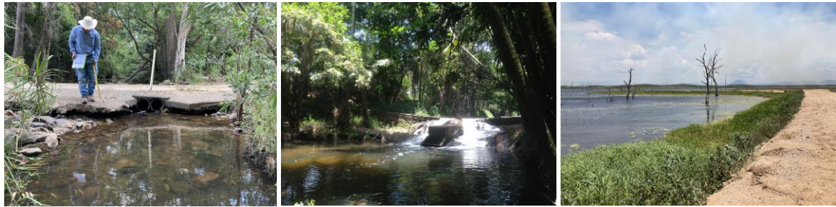
Figure 10. Examples of typical fish barriers validated during ground truthing. Road causeway - left, weir - middle and bund - right.
