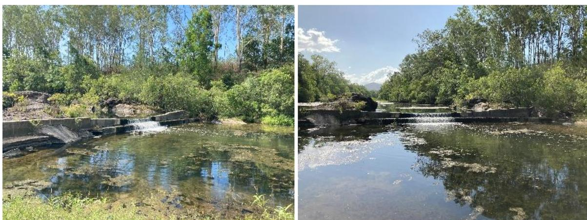
**Figure 16. The Andromache R gauging weir under low flow conditions.**
