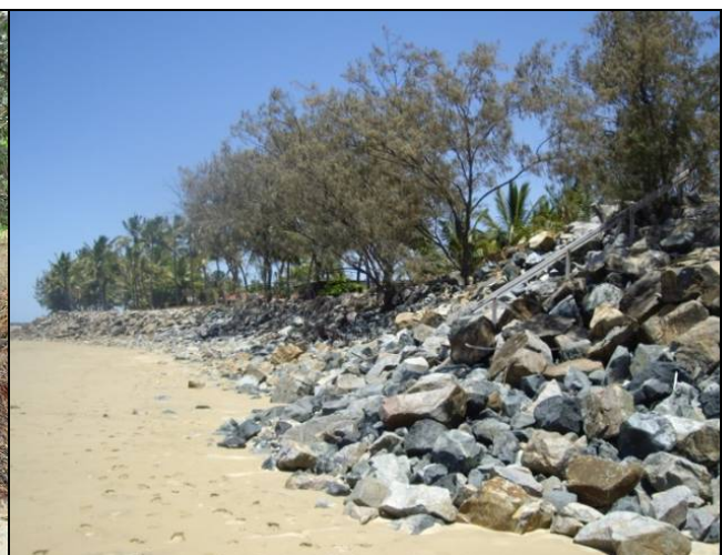
Figure 16: Rock walls have been erected along portions of Mackay beaches to combat erosion.
