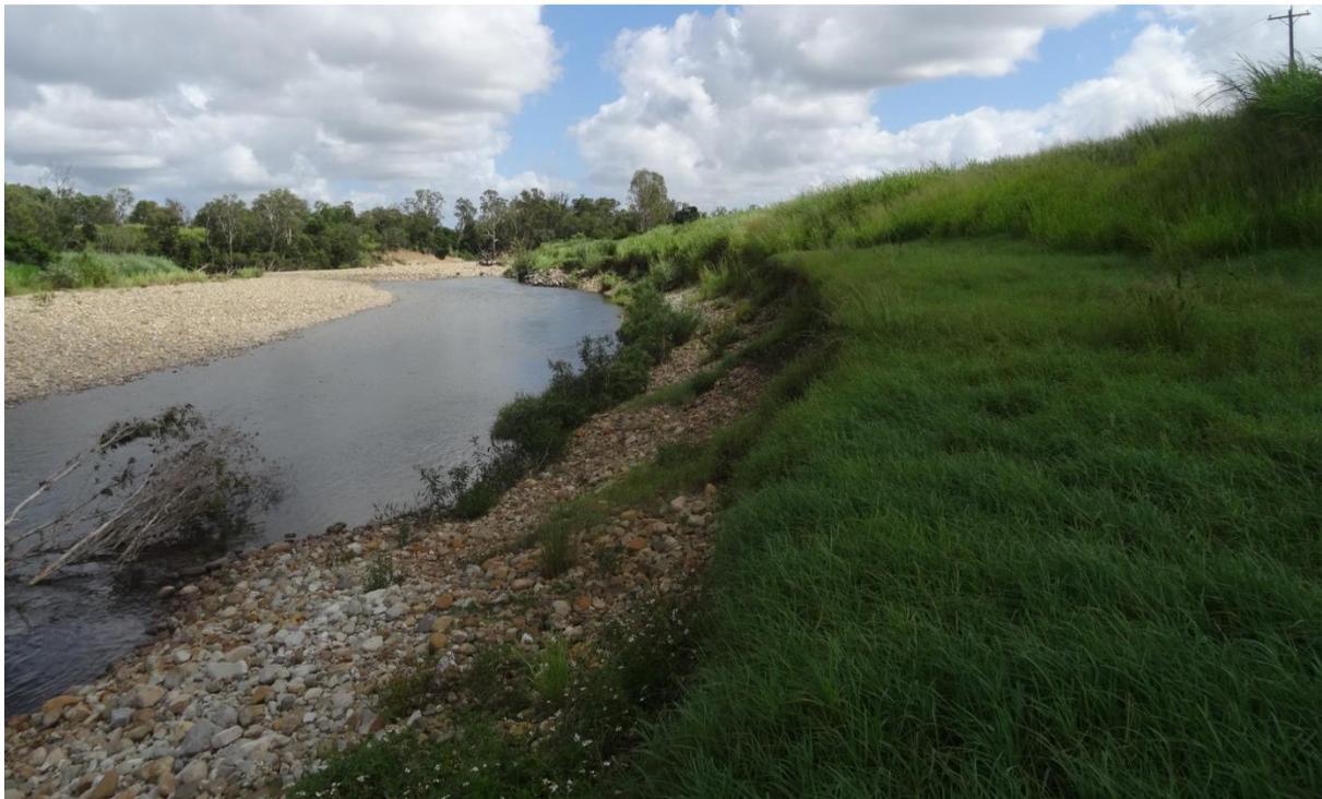
**Figure 24.** Looking downstream along the right bank located 1.5 km upstream of the Boundary Creek confluence. Site is subject to meander migration. This site has contributed 3,000 m<sup>3</sup> of sediment loss between 2010 and 2014.
