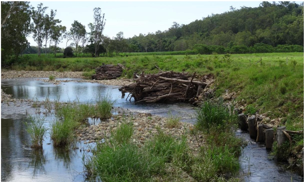
**Figure 36.** Engineered Log Jams near the upstream extent of Reach 4
