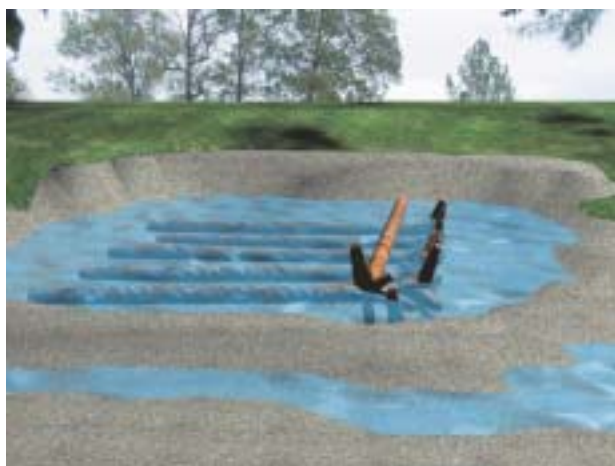
Step 4. Place first cross spanning log.
