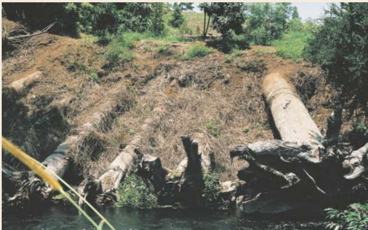
Photo 8. Early model log bank revetment, with cable and rock ballast — Obi Obi Creek, Queensland.
