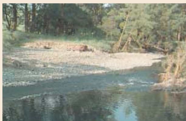
Photo 35. Bank deflector jam that appears to have failed, but in fact is still there — only buried. This is a case of the structure being over designed and too effective — to the extent that it initiated so much deposition that the whole structure was buried and the channel shifted laterally by ~20 m. In this case the structure is still performing its primary engineering role — even while buried. It provides woody substrate in the hyporheic zone, and a source of slow release carbon to the system. In this instance we may need to reconsider what is meant by “failure”.
