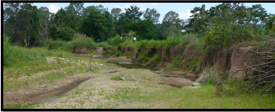
Figure 2 Looking upstream from bed at left bank where Reef Catchments revegetation works have been lost to erosion.
