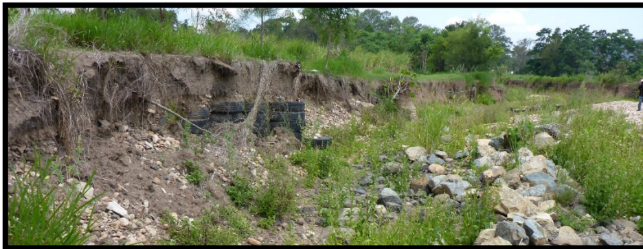
Figure 1 Looking downstream from bed at left bank where Reef Catchments rock toe protection works have been outflanked.
