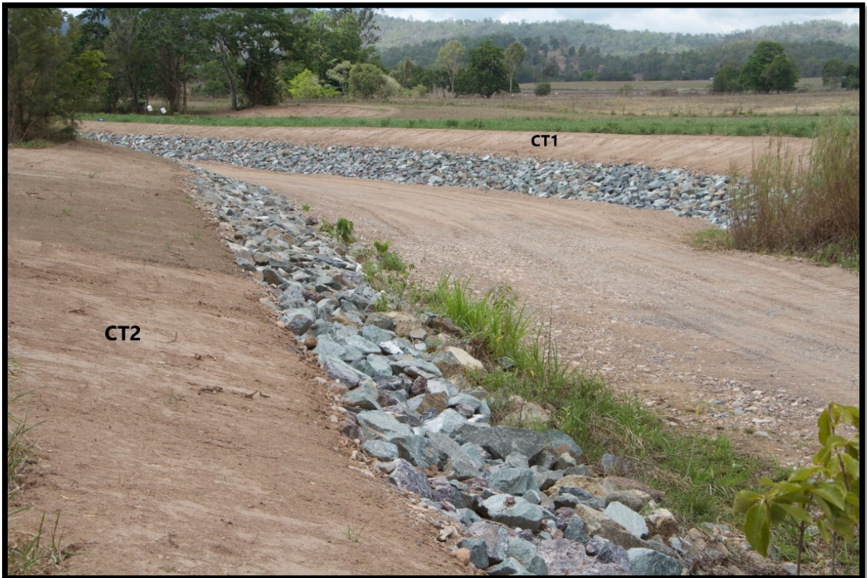
Figure 5 CT1 & CT2 Post Earthworks (Pre Planting)
