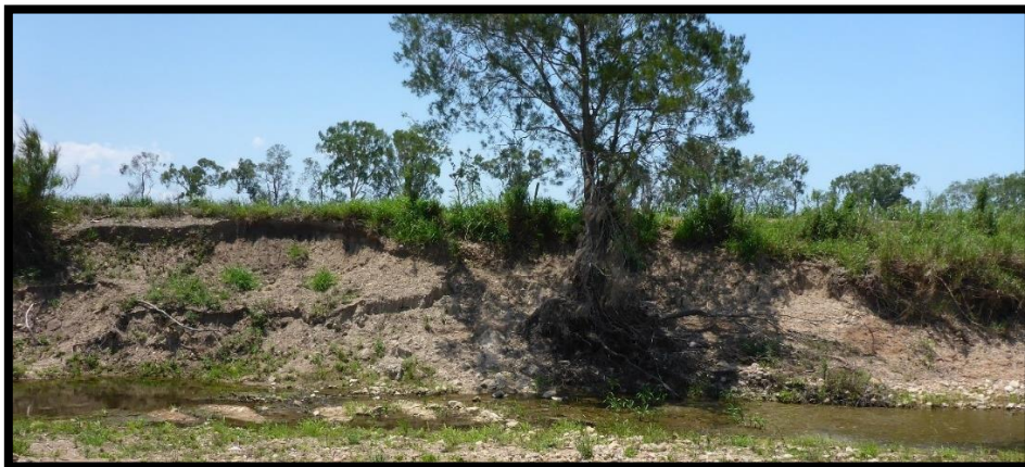
Figure 1: Erosion at WH1, Nov 17
