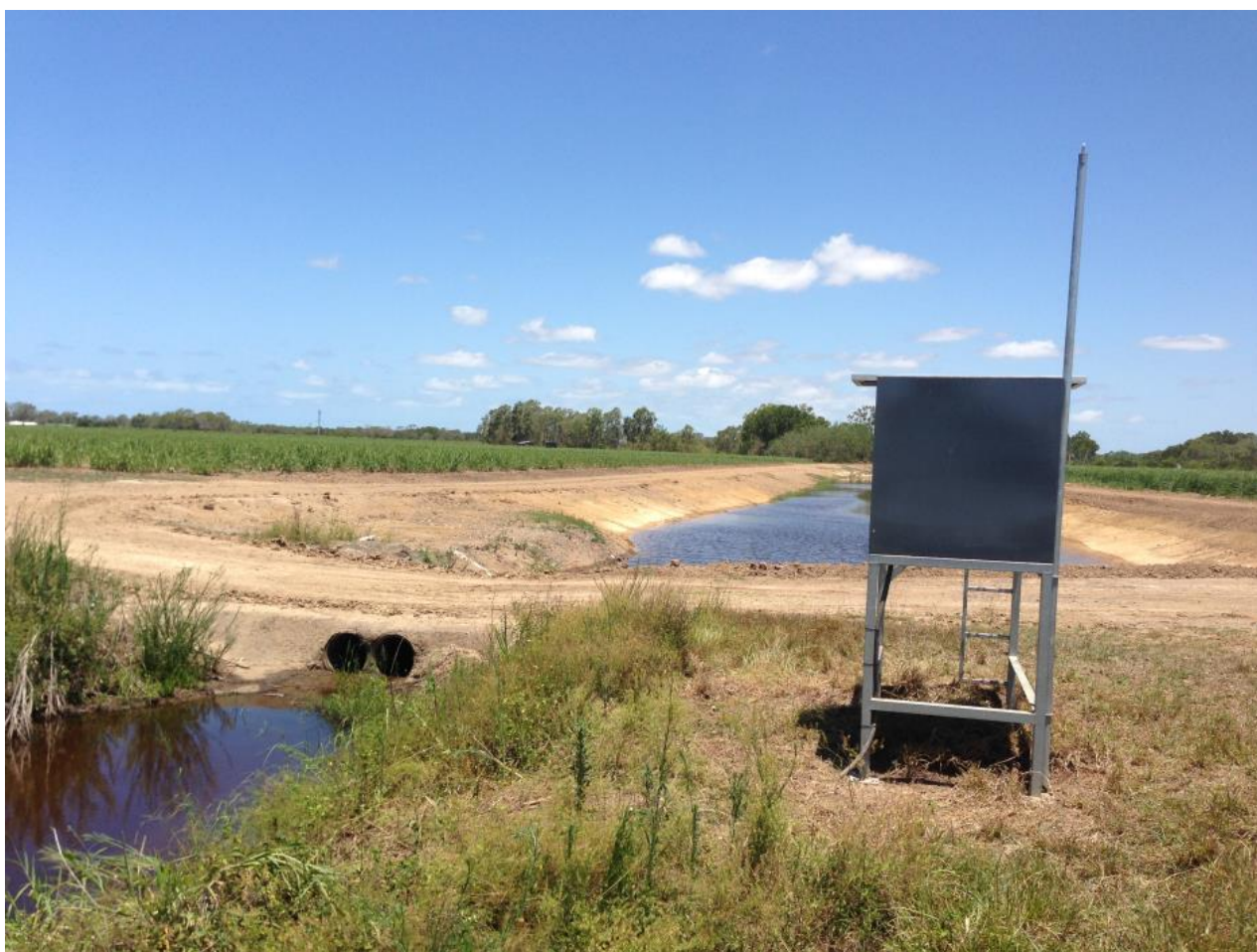
Figure 5 The bare, battered banks are a possible cause of increased sediment concentrations at the outlet (looking downstream from the inlet sampler, along the sediment basin)
