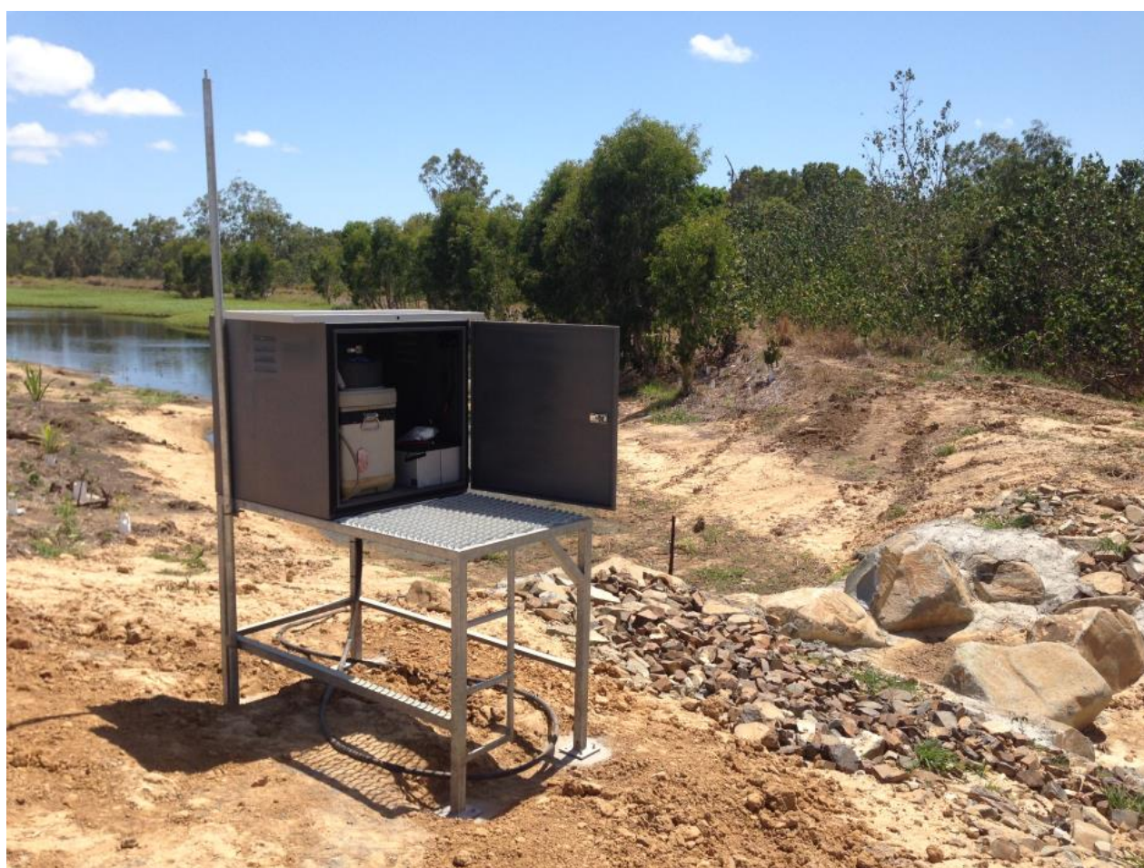
Figure 3 Water quality sampling equipment at the outlet of the Bakers Creek system repair site, showing the ISCO Avalanche sampler in the grey enclosure. The float switch is attached to the star picket in the centre of the photo.
