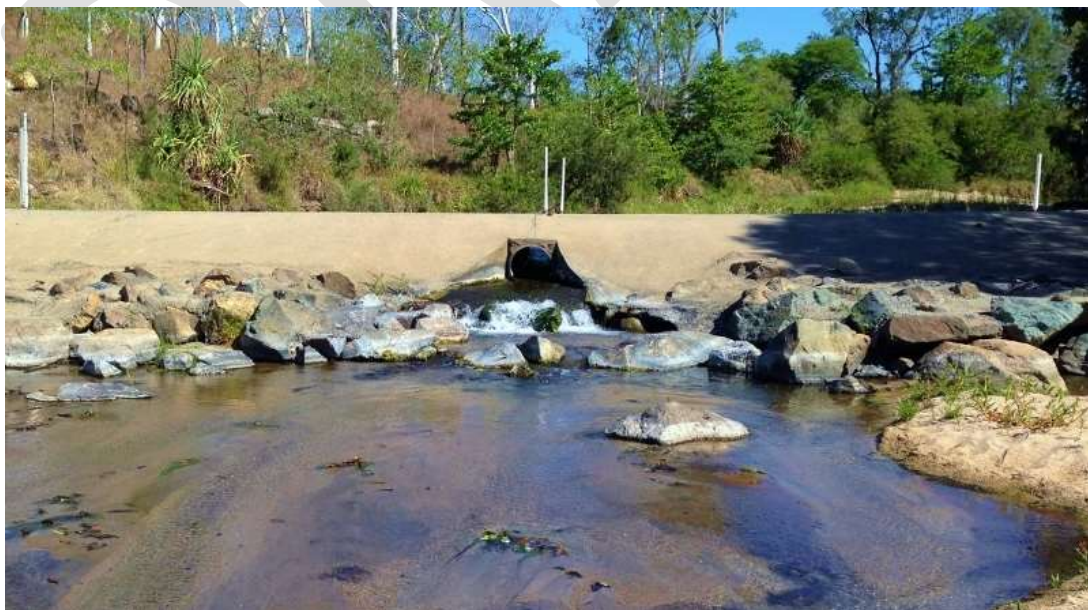
Figure 4. One of only two barriers located on 'Major' and 'High' impact streams within the Andromache sub catchment; 1 pipe causeway on the perennial Mares Nest Creek. This causeway acts as both a 'velocity' and 'water surface drop' barrier to fish migration.
