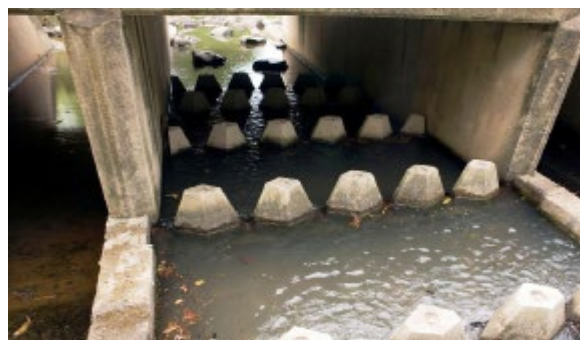
The pre-cast concrete cone fishway installed on Seaforth Creek has helped restore critical fish passage and flow in the Constant Creek catchment management area
