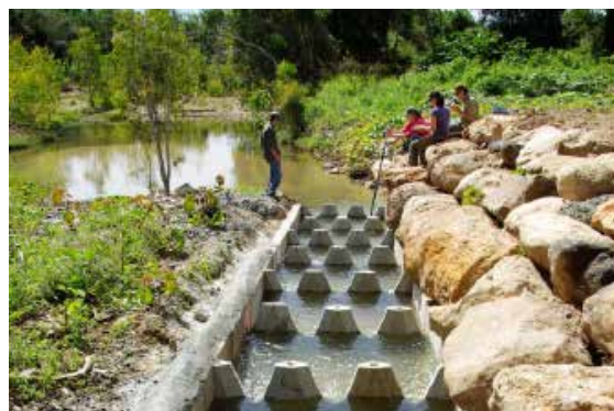
Pre-cast concrete cone fishway installed on Flaggy Rock Creek to reinstate critical passage and flow for fish migration.
