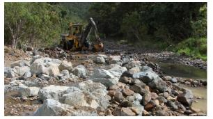
Construction of a rock ramp fishway in the upper reaches of the Gregory River removed a critical barrier to fish migration
