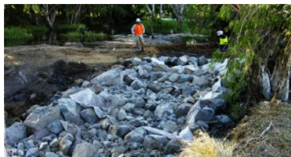
A key barrier to fish migration has been removed with the construction of this rock ramp fishway on Lethe Brook
