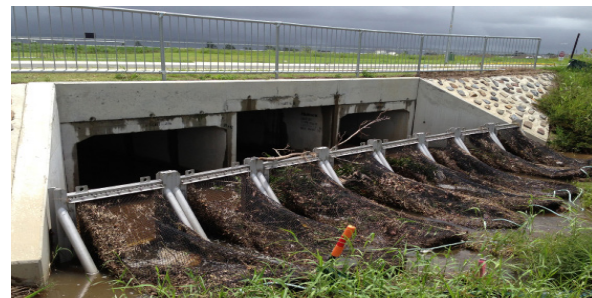
Gross pollutant stormwater trap installed at Paget as part of a management program that includes monitoring the type and quantity of debris collected from industrial and urban areas
