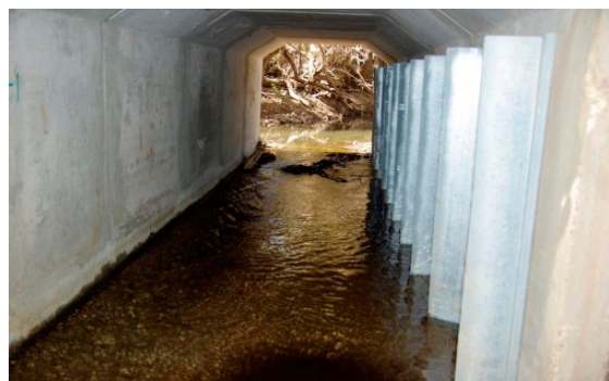
The culvert baffle fishway constructed on Marion Creek helping to restore critical fish passage and flow .
