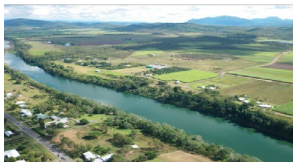
Pioneer River Main Channel showing intensive production land and rural urban development adjacent to a narrow riparian margin.
