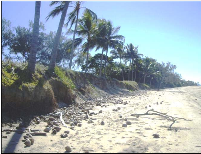
Figure 26: Some sections of the frontal dune along Seaforth Beach are lacking native vegetation, leaving them vulnerable to erosion processes.
