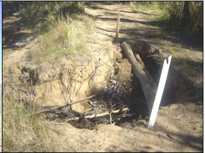
Figure 27: Inappropriate vehicle access has resulted in localised erosion.
