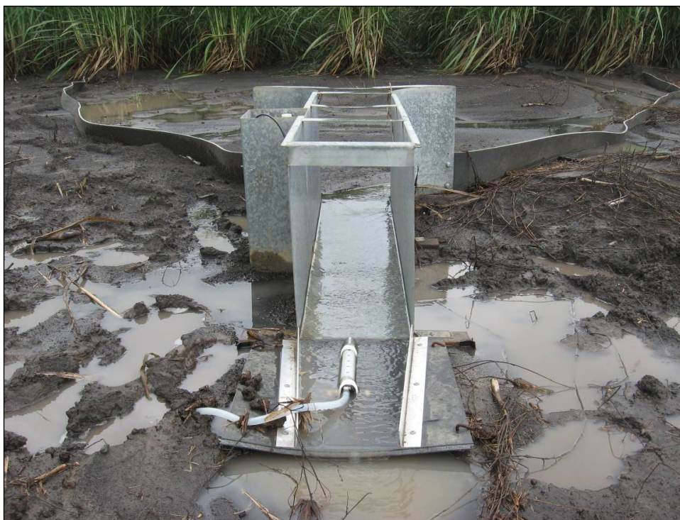
Figure 7. Example of a flume installed at each strip scale monitoring site.
