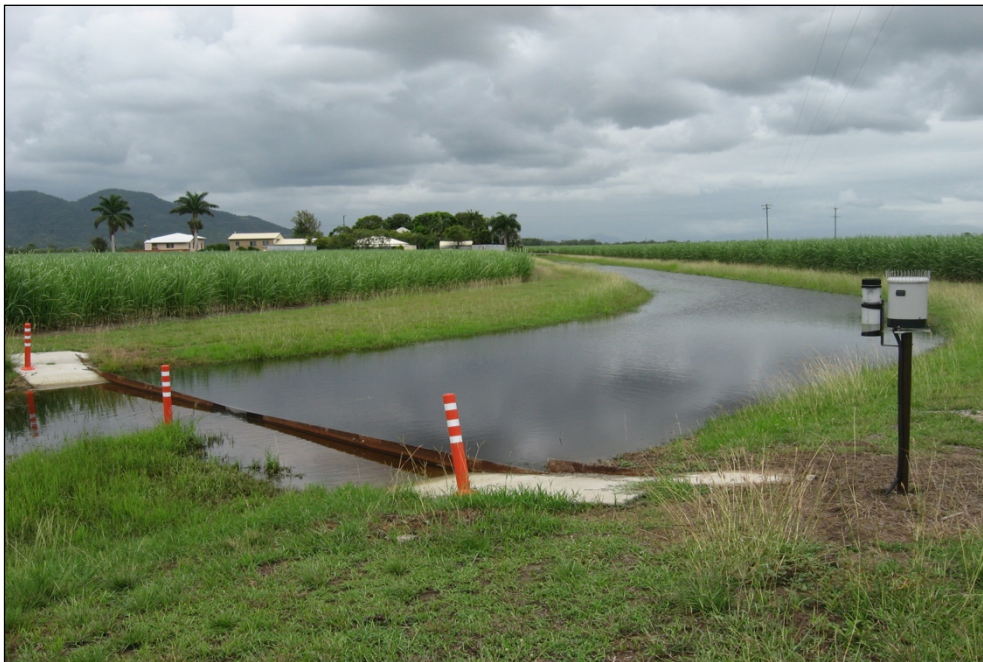
Figure 4. V notch weir located at the multi-block scale monitoring site.
