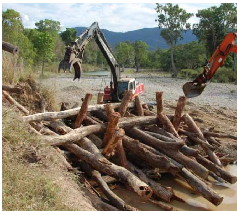
One of three engineered log jams on the O'Connell River.
