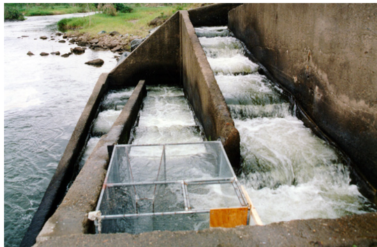
Figure 3. Northern Hemisphere designed pool and weir fishway on Marian Weir (Pioneer River, QLD). Excessive turbulence and velocity produced by this ‘fishway’ acts as a barrier to most Australian native fish.
