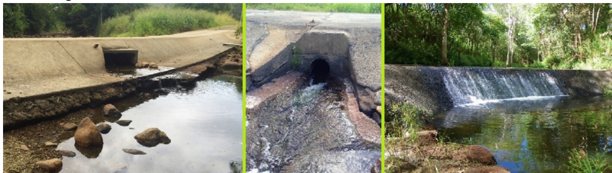
Figure 4. Left to right: Culvert causeway (Patullo Road, Gregory River) displaying a water surface drop, shallow water surface (through culvert and on apron) and velocity barrier (during medium-high flow conditions) exacerbated due to a culvert diameter <60% of stream width; Blackrock Creek pipe causeway displaying velocity and behavioural barriers (dark shadows/insufficient lighting in pipe) and water surface drop barrier (Sandy Creek Tributary).
