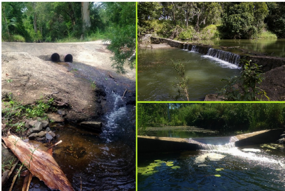
Figure 2. Different barrier types: pipe culverts and concrete apron (downstream) (left); weir (top right) and V-notch gauging weir, (bottom right).
