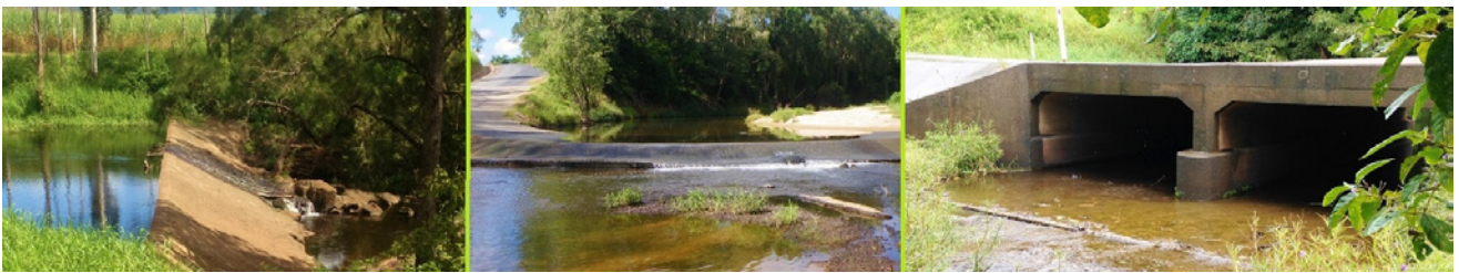
Figure 5. Left to right: Low transparency barrier (Macquarie Ck Weir), Medium transparency barrier (Palm Tree Rd causeway, Sandy Ck), High transparency barrier (Myrtle Ck).
